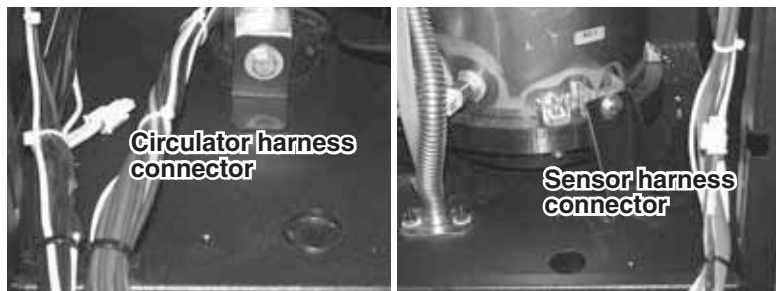
Figure 15 WM97+155 harness connector locations
