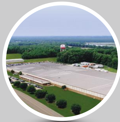
400,000 sq. ft. production, engineering, manufacturing facility
