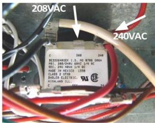
If the line voltage being supplied to the electric furnace is 208-volt single phase, the line voltage tap on the low voltage transformer needs to be moved from the 240-volt tap to the 208-volt tap. If this is not done, the secondary output voltage of the transformer will be too low.
