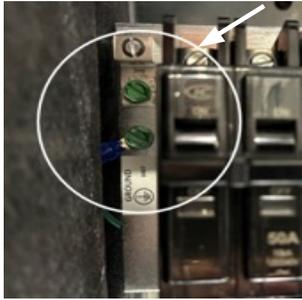
Line voltage wiring should be routed through the access holes at the top of the electric furnace. Proper electrical conduit connection fittings should be used. Connect the power wiring to the line side connections on the electric furnace. The electrical ground wire should be connected to the grounding lug. Ensure both the field supplied ground wire and electric furnace GREEN ground wire are both secured to the grounding lug of the electric furnace.
