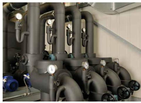
Armacell's newest innovation, ArmaFlex Ultra with FlameDefense™ Technology, is the **first** elastomeric foam insulation Classified by UL to UL 723 at 25/50. This third-party certification proves our commitment to product safety and compliance. All AP ArmaFlex-branded products are made with Microban® antimicrobial protection, are GREENGUARD Gold certified and now have Environmental Product Declarations (EPDs) to show our dedication to material transparency.
