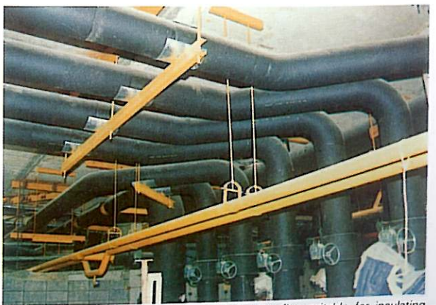
Many advantages as described above, make Aeroflex suitable for insulating chilled water piping.
