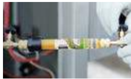
Charge inline with refrigerant
