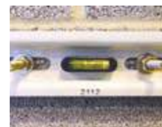
Built in wall bar spirit level
