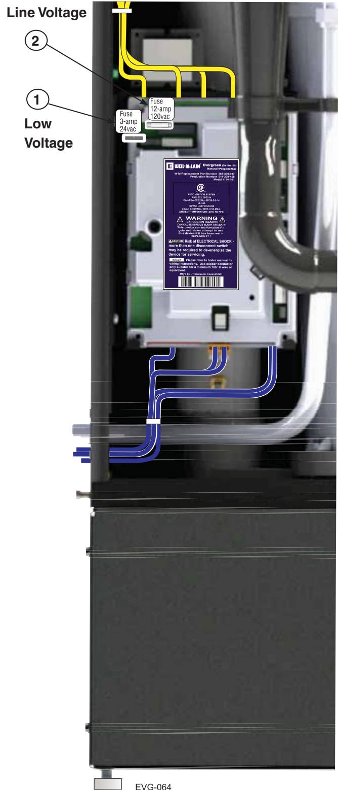
Figure 93 Control fuses
