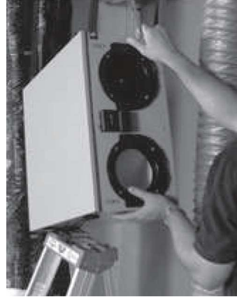
Figure 6.2 Pull on the middle strap and gently push upward on the unit. Then repeat procedure on the other side.
