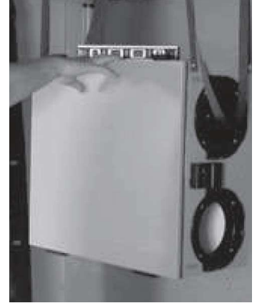
Figure 6.3 When completing the procedure make sure that the HRV or ERV is leveled
