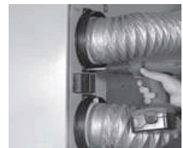
Figure 7.5 Fix and secure with two screws supplied
