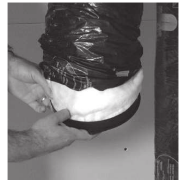
Figure 7.2 Insert insulation inside the collar.
