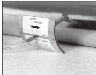
Inserting Air flow grid in duct
