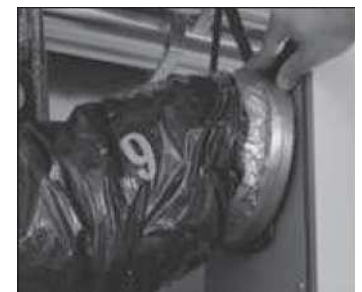
Figure 7.4 Slide collar on the unit
