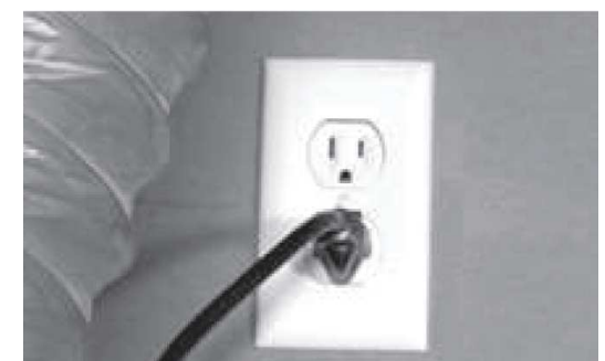
Figure 9.2 It is recommended that the HRV or ERV have a dedicated receptacle with 115v. It is not recommended to connect unit with an extension cord. If no receptacle is available, please call an electrical contractor and have one installed. Insure polarized plug is correct.
