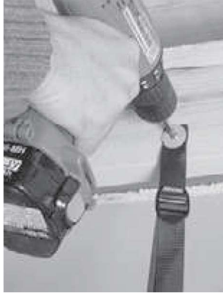
Figure 6.1 Attach your four straps to the floor joist making sure that you attach thru the washers and the grommets
