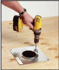
Mount SureGrip support plate.
