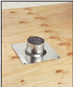
Push pipe through vent support.
