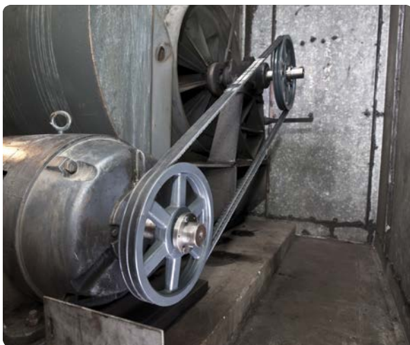
Browning Optimized 2 groove 5VX Solution
